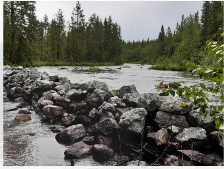
The oldest cleared rapids were entirely cleared by hand, involving hard work where watercourses were manually cleared, and the material was thrown up to form embankments. Later, stump extractors started being used to lift larger blocks. Eventually, the work was mechanized with excavators and bulldozers.
